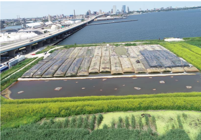
Geotubes at Port Milwaukee that contain removed sediment.
